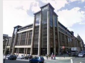
Exchange House, Glasgow
