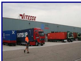
Venlo Logistics Centre, Venlo
